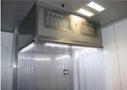
Ceiling Laminar Airflow units protection against contamination which EN ISO 14644-1 ) as well as to pharmaceutical industry provide enhanced aseptic work zones by utilizing unidirectional airflow to positively pressurize and purge the working environment from contaminants , CLAF • Modular easy to clean design , Zoned Magnehellic gauges for filter loading , PVC Curtains ,
